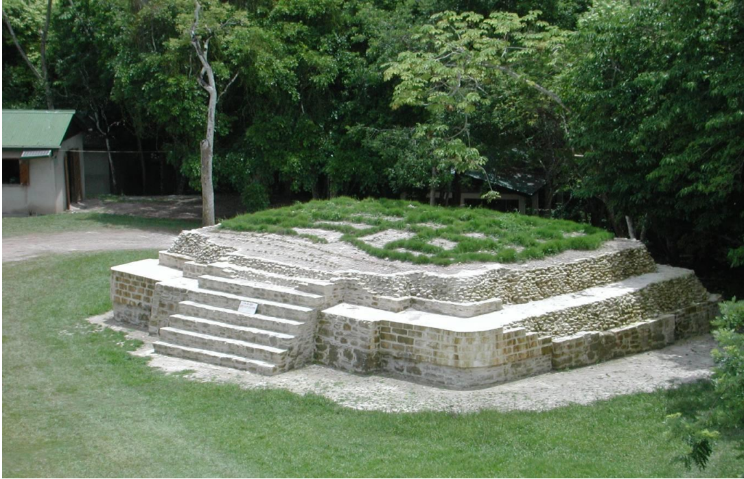
Figure 28. Photo of Structure A14 after the TDP excavation and conservation (photo by J. Awe, courtesy of BVAR).
